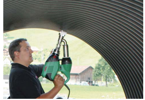
The handy WELDPLAST S2 welding vertically.
