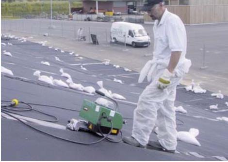
The COSMO in use on a landfill covering.
