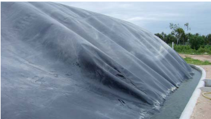
Gas extraction plant in Austria
