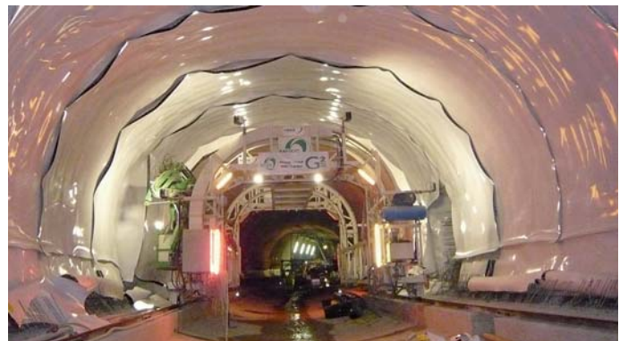
Tunnel construction in Germany
