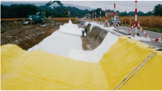
Geomembranes in road construction, Switzerland
