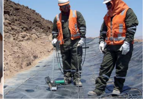
TWINNY S with combi-wedge, welding in a South American mine.
