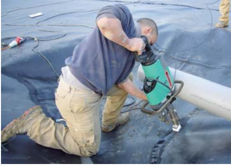
WELDPLAST S6 undertaking assembly applications on a landfill site.
